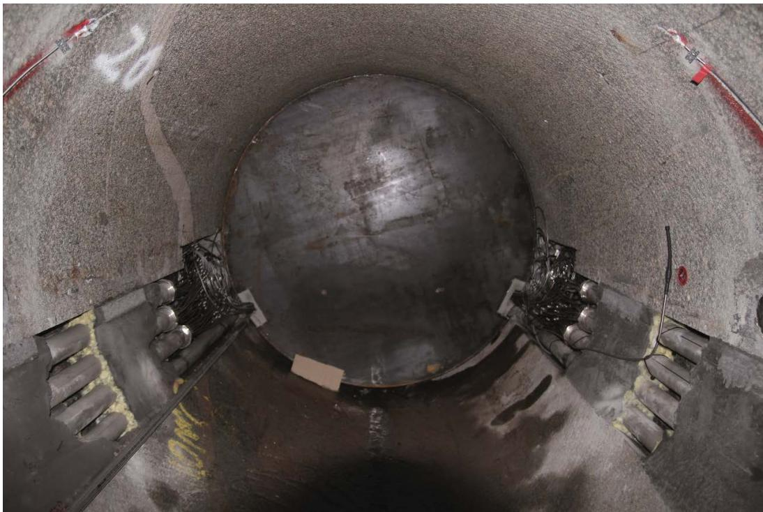
**Figure 5-10.** Supercontainer positioned in the drift with all its cables pulled. The tight fit between the supercontainer and drift wall is clearly visible. A small paper has been placed down to the left of the supercontainer to ensure that the deposition machine will detect the supercontainer during deposition of the next component.
