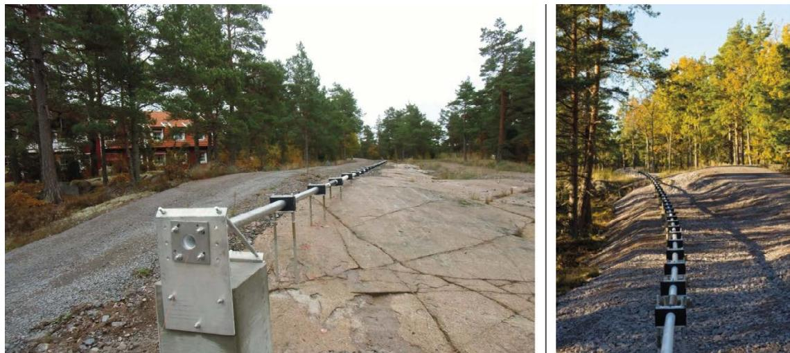
**Figure 4-7.** Äspö deviation control facility is a 300 m long plastic tube ( $\varnothing 75$  mm) secured firmly to the ground with 151 fastening devices. All material used in the construction is non-magnetic such as plastic and aluminium (Nilsson 2015, Figure 4-1).
