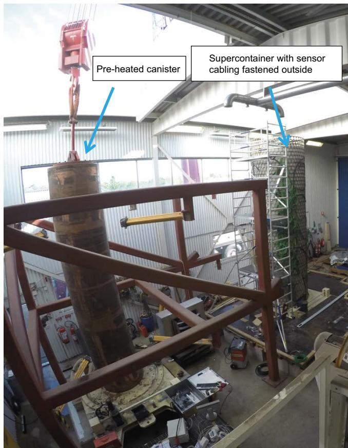
**Figure 5-17.** Pre-heated canister being prepared for installation inside the supercontainer.
